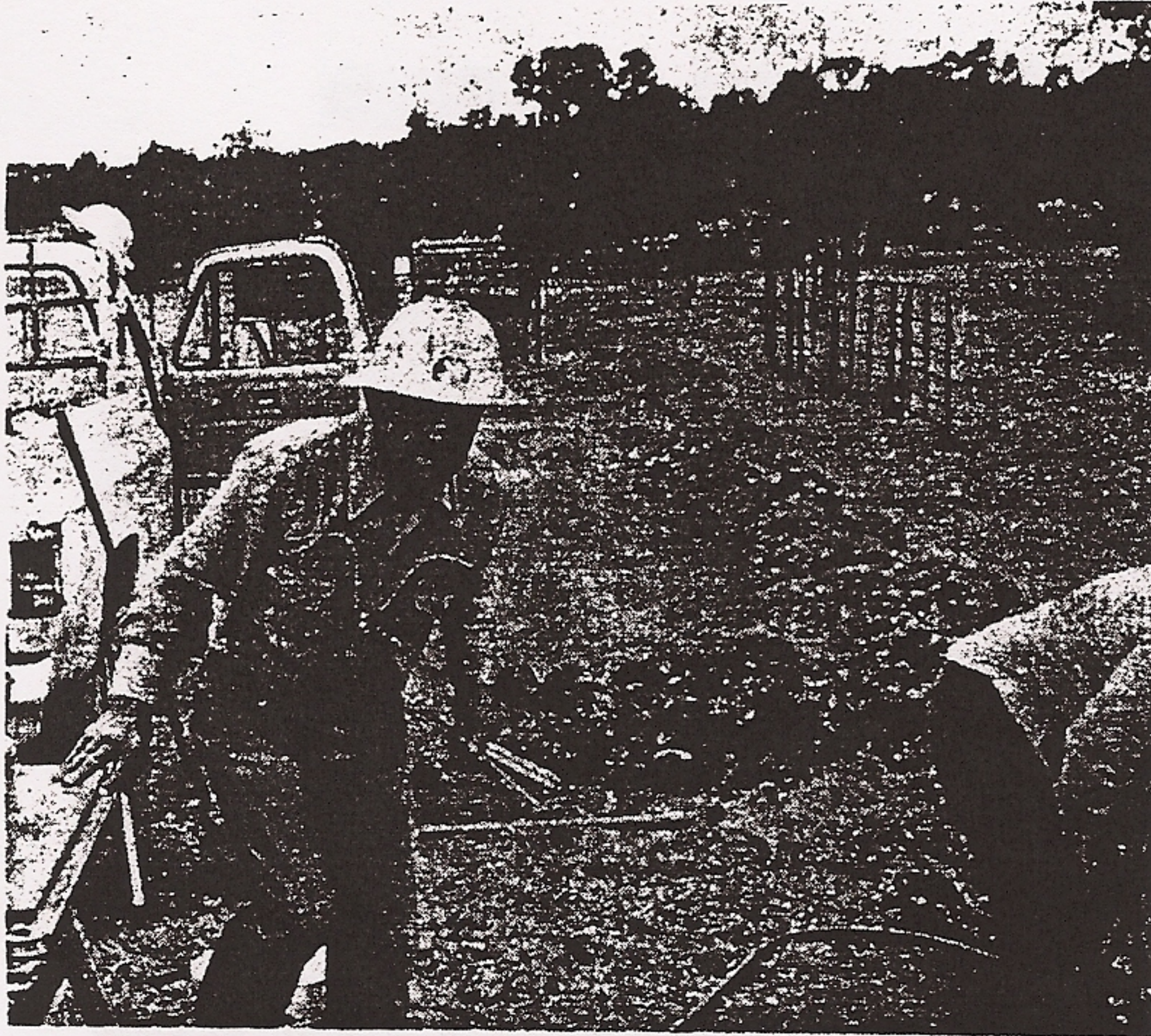
BUILDING a new corral
